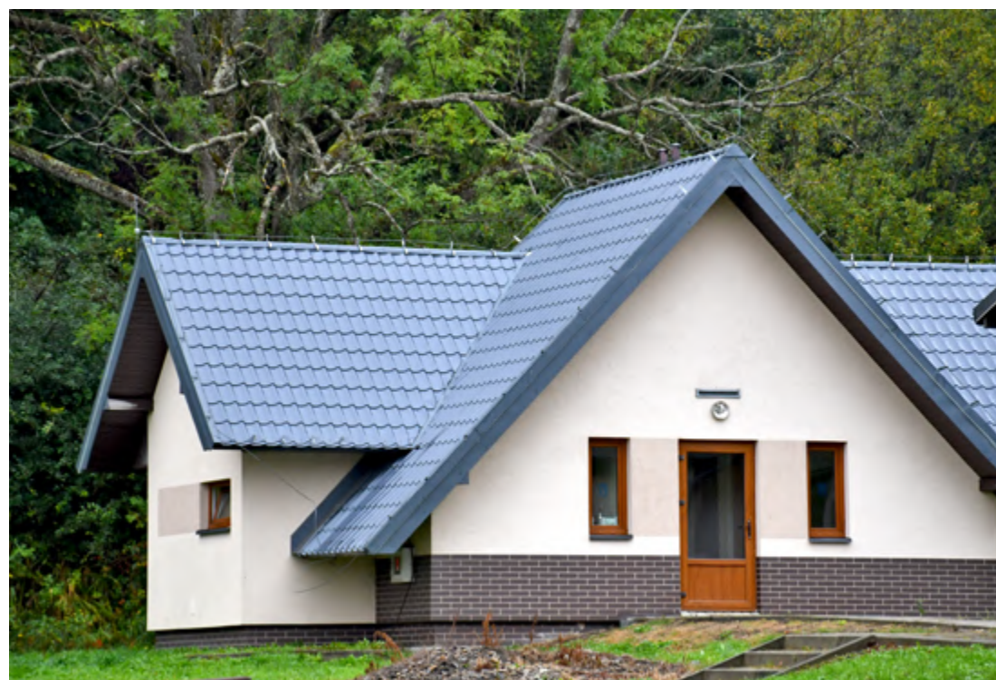
Wetlina - zaplecze kuchenne przy remizie OSP Wetlina - kitchen facilities at the fire house
